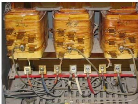
Overheated dry transformer – C phase (visual and thermal images) Photo Source: Predictive Service
