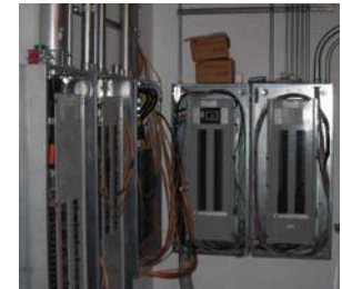
Combustible debris with dry Transformer housing Photo source: Predictive Service
