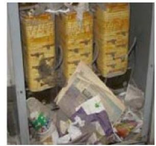
Combustible debris with dry Transformer housing Photo source: Predictive Service
